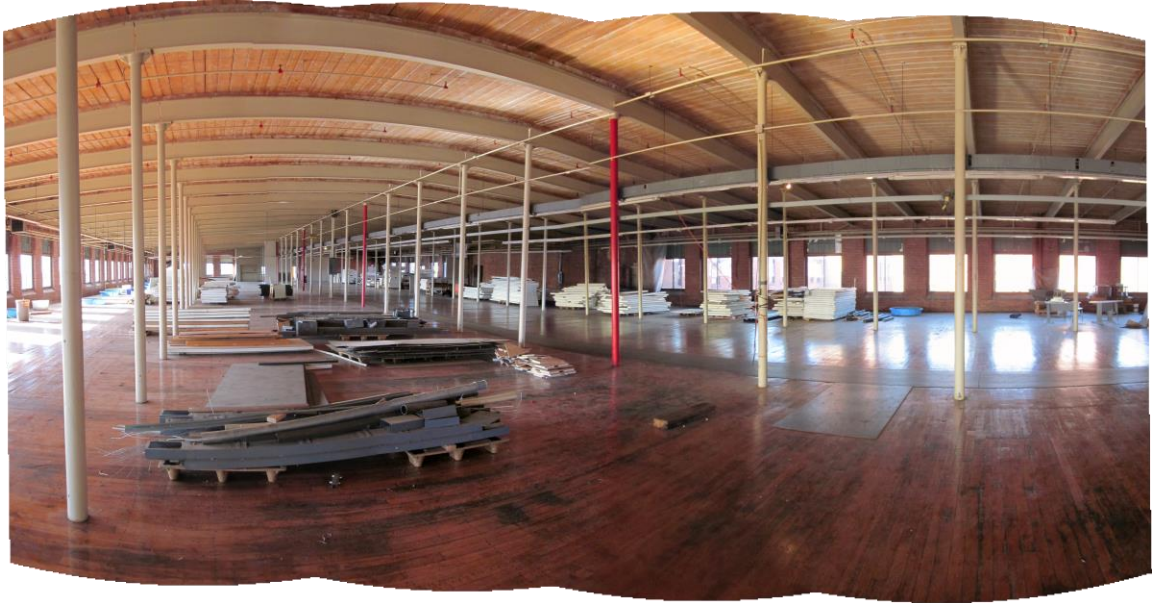
Figure 5: A floor in the Open Square Building in Holyoke, Massachusetts
